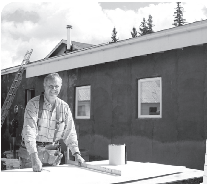
Retrofit Project Lead, Karl Monetti, custom cuts pieces of insulating foam for the exterior retrofit. © Laenne Thompson
