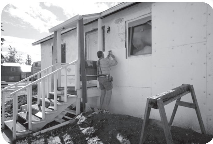
Above: Insulating foam is applied. © Laenne Thompson, Right: Karl Monetti stuccos the front of the building. © Pamela A. Miller
