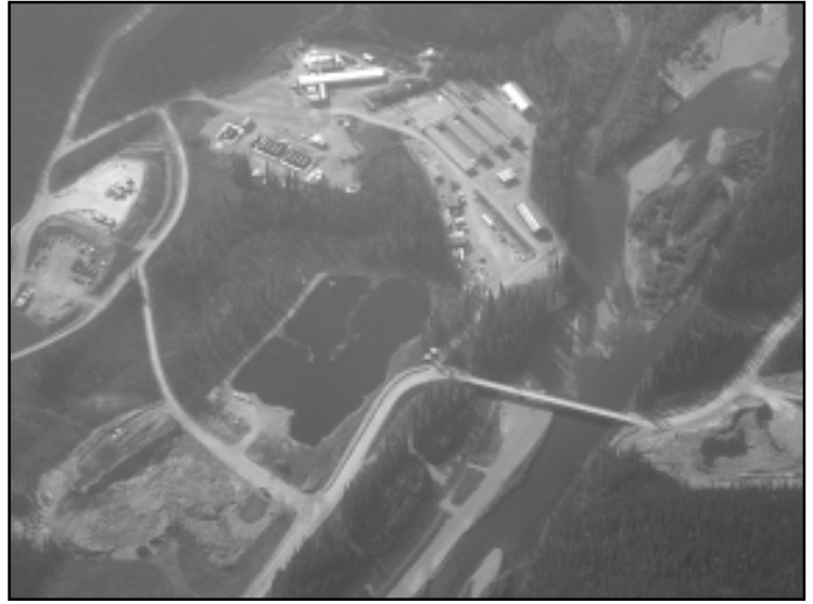
Pogo mine site with Goodpaster Bridge in August 2004. © NAEC.
