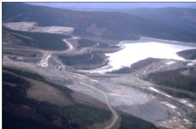
The tailings impoundment at the Fort Knox Gold Mine, where 1,177 acres of the Fish Creek drainage were converted to a waste treatment facility. NAEC file photo.
