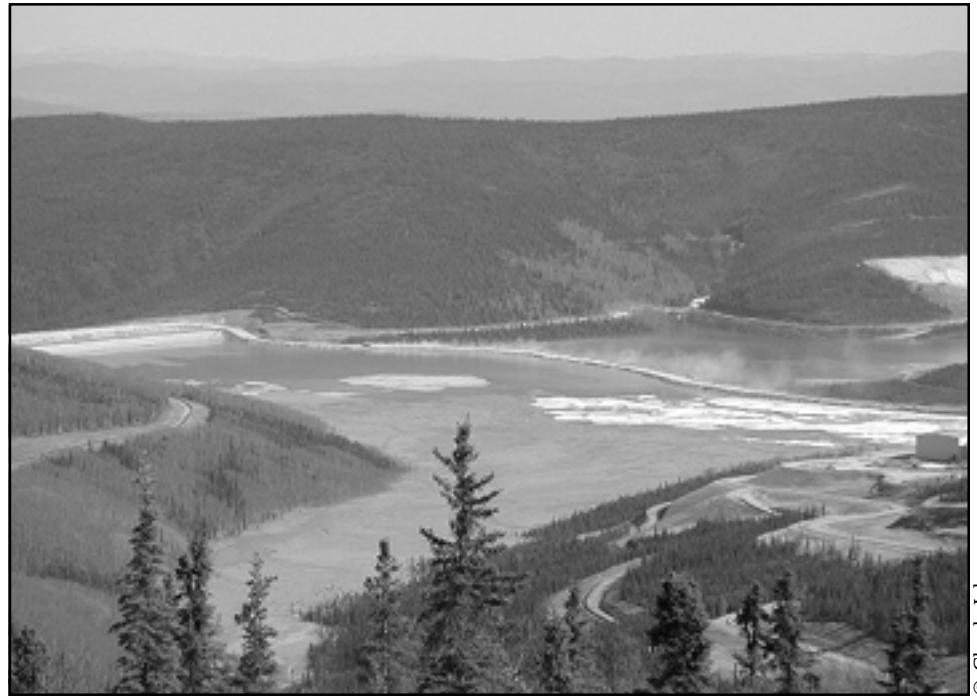
Ft. Knox tailings impoundment.
