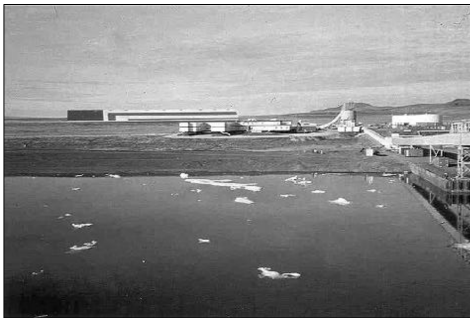
Concentration storage barn at the Delong Mountain Terminal, northwest Alaska.
