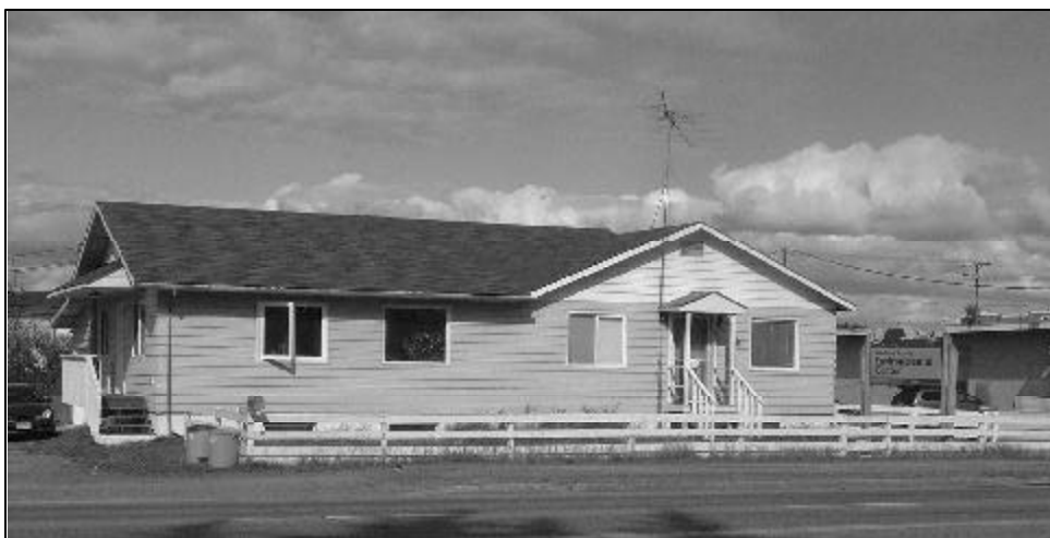
The offices of the Northern Alaska Environmental Center, located on College Road in Fairbanks, recently underwent an "energy audit" to determine the energy efficiency of the building.
