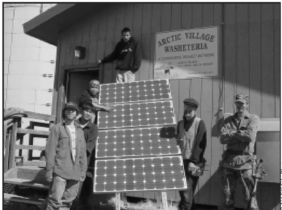
Residents of Arctic Village shared a sense of community and activism while they installed solar panels throughout the village.
