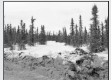
On January 20, Fairbanks Gold Mining began clearing the road for the True North mine.
